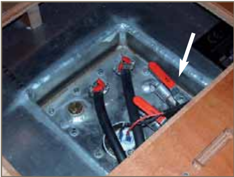
ENGINE FUEL VALVE
