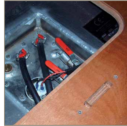
FUEL VALVES FOR ENGINE AND GENERATOR
