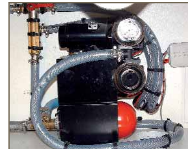
PRESSURIZED WATER PUMP
