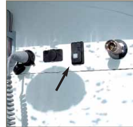
DECK WASH PUMP SWITCH
