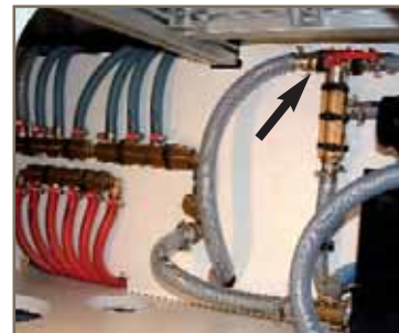
TANK SELECTION VALVE + MANIFOLD
